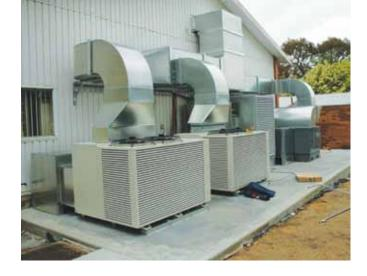
Above and left: The return air / outside air mixing plenum has large capacity air intake bag filters that are housed behind a louvre door, making service easy.
